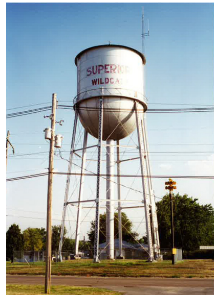
Superior water tower. 2000 photo.
