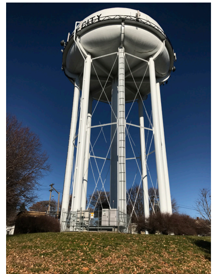
Nebraska City water tower.
