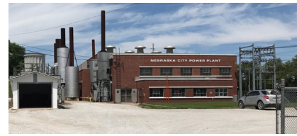
Nebraska City power plant.
