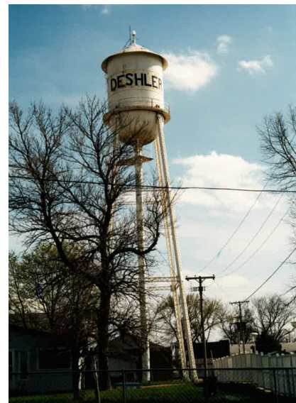
Deshler water tower. 2001 photo.
