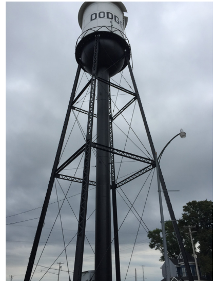
Dodge water tower. 2016 photo.
