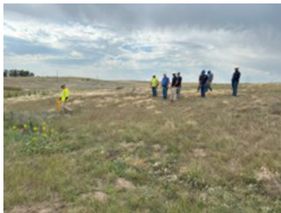
Jim Meyer of Wesco instructing linemen how to locate primary and secondary conductors.
